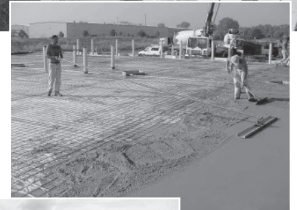
To finished floors and curbs...
