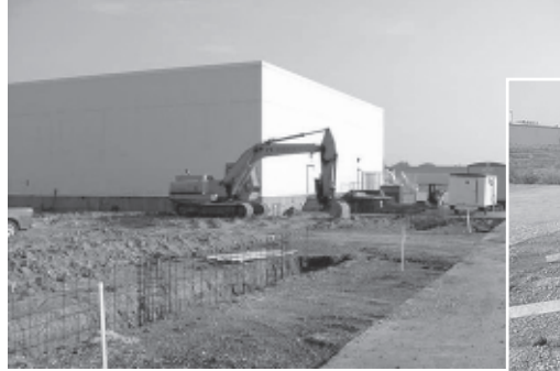
Starting from the ground work...
