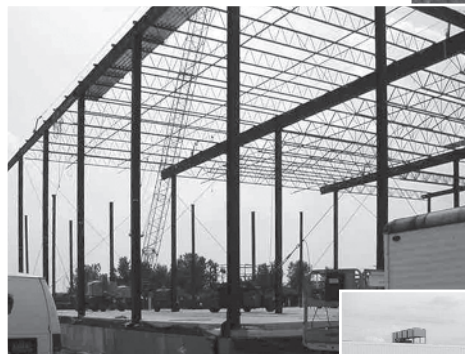
To the steel superstructure...
