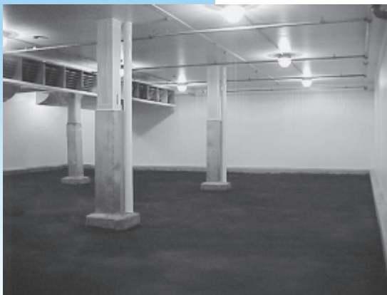
Another successful renovation! Before and after...
